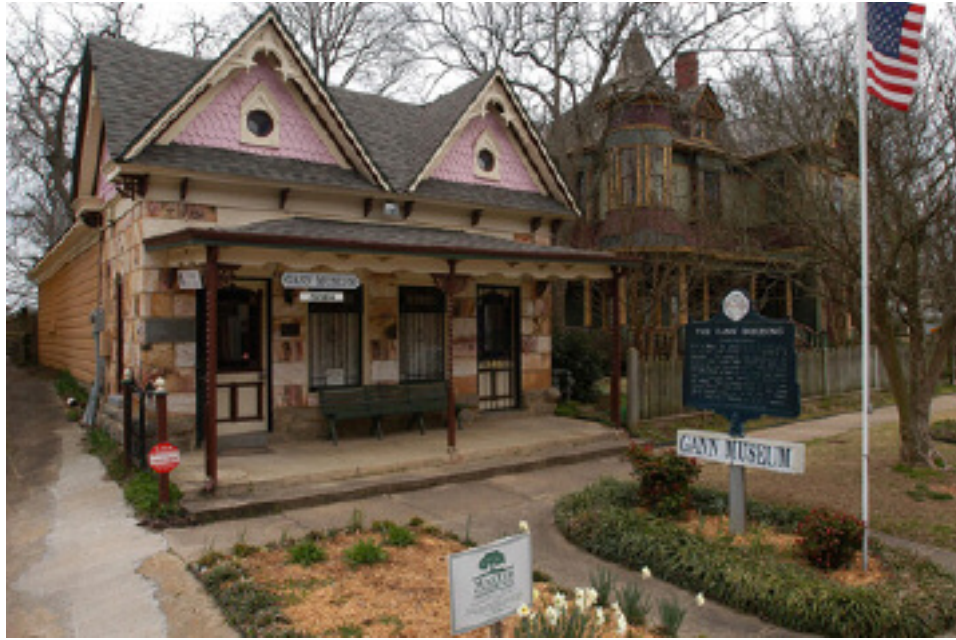
The Gann Museum in Benton commemorates the town's bauxite mining history – starting with this distinctive building, the only known structure in the world made entirely out of bauxite.
